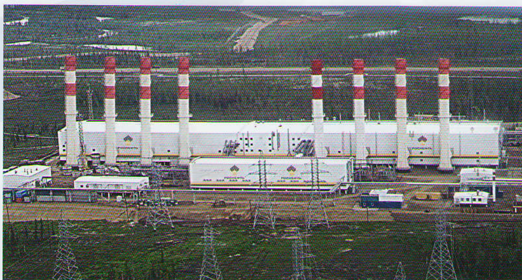
8 waste heat boilers (KUV-33) after 8 General Electric MS-5001 (26 MW) at 200 MW power plant, Vankor Oil Field, Russian Federation
