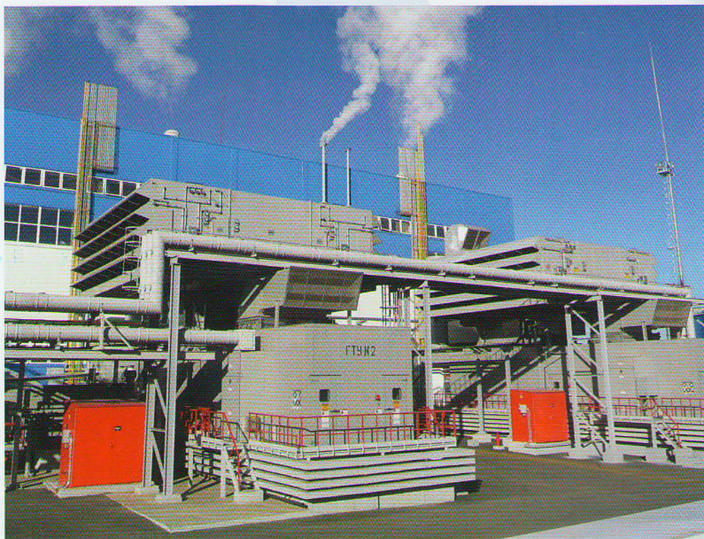
2 HRSGs (KUP-75-3.9-440, 75 t/h of steam) after 2 General Electric LM6000 PD Sprint (45 MW) at 115 MW CHP plant, Voronezh, Russian Federation
